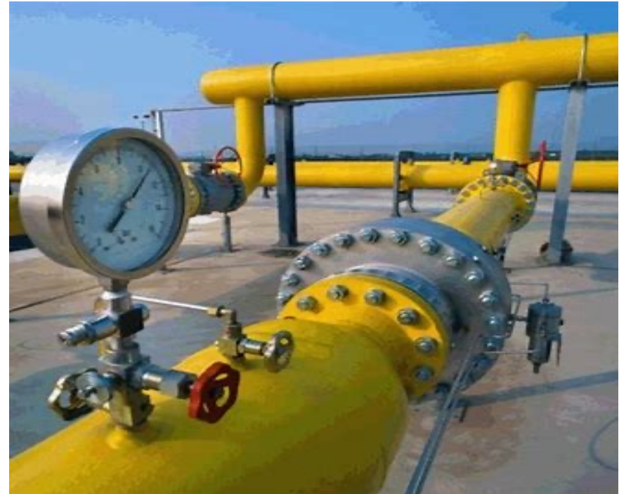
Pneumatic pressure testing
